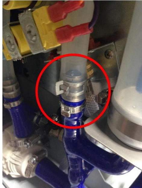
Connect the condensate hose
